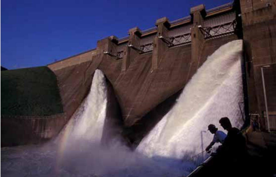
Kinzua Dam Warren County
